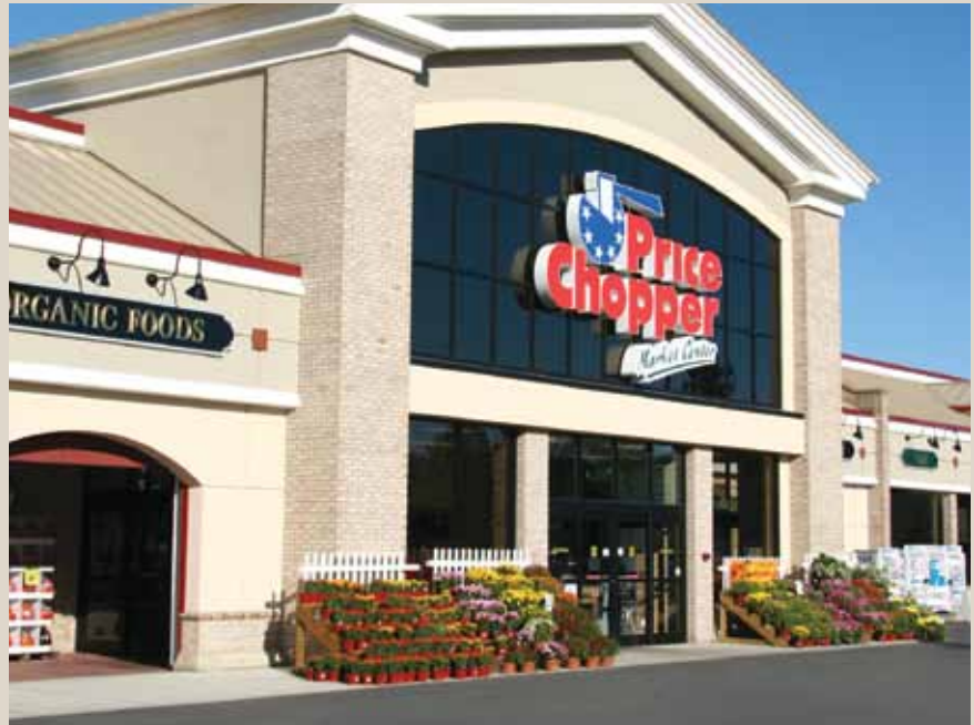
The Malta, NY, store location is a greener supermarket as a result of significant efficiency upgrades to its refrigerated foods section.
