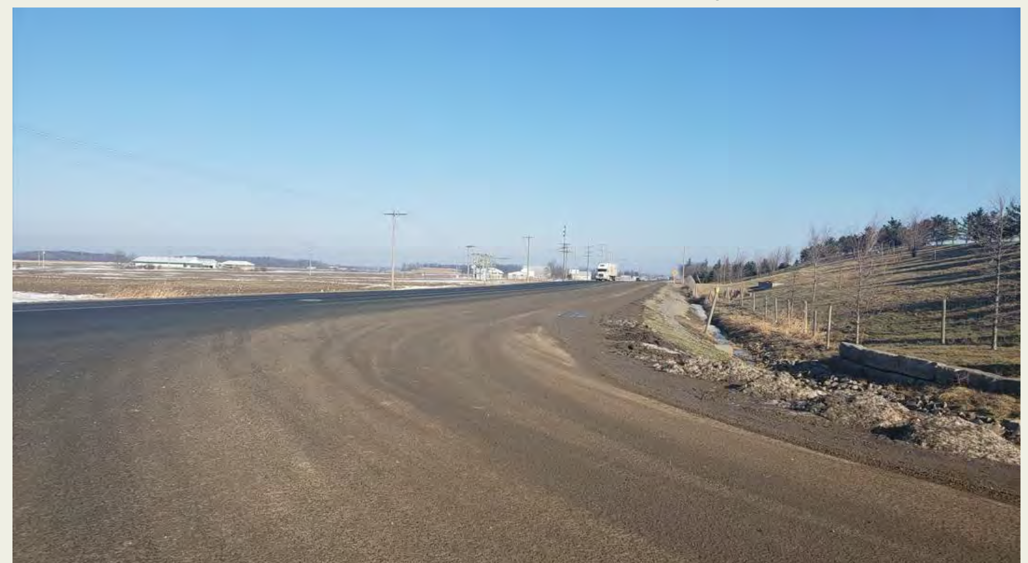
TCEC Driveway at Nauvoov Road Looking North
