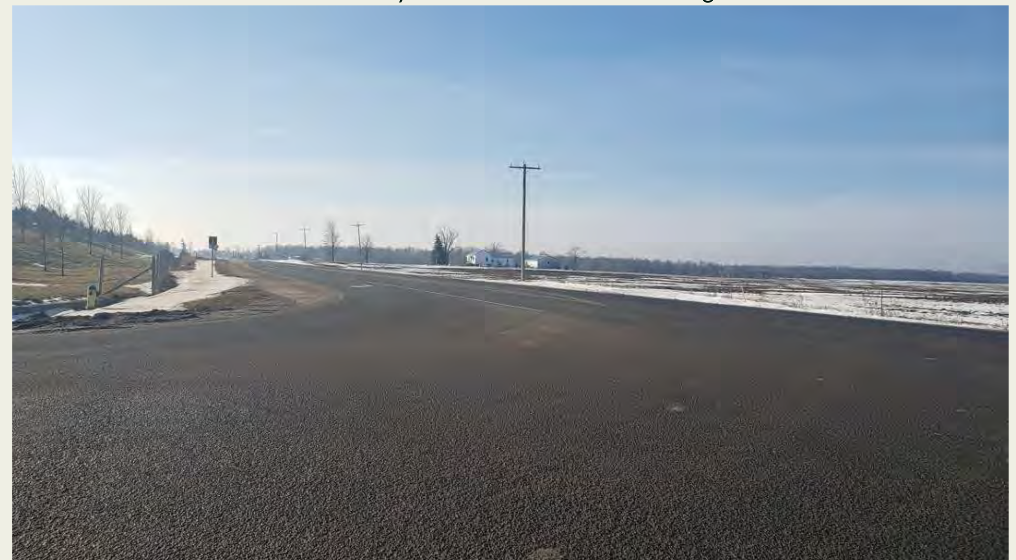
TCEC Driveway at Nauvoov Road Looking South
