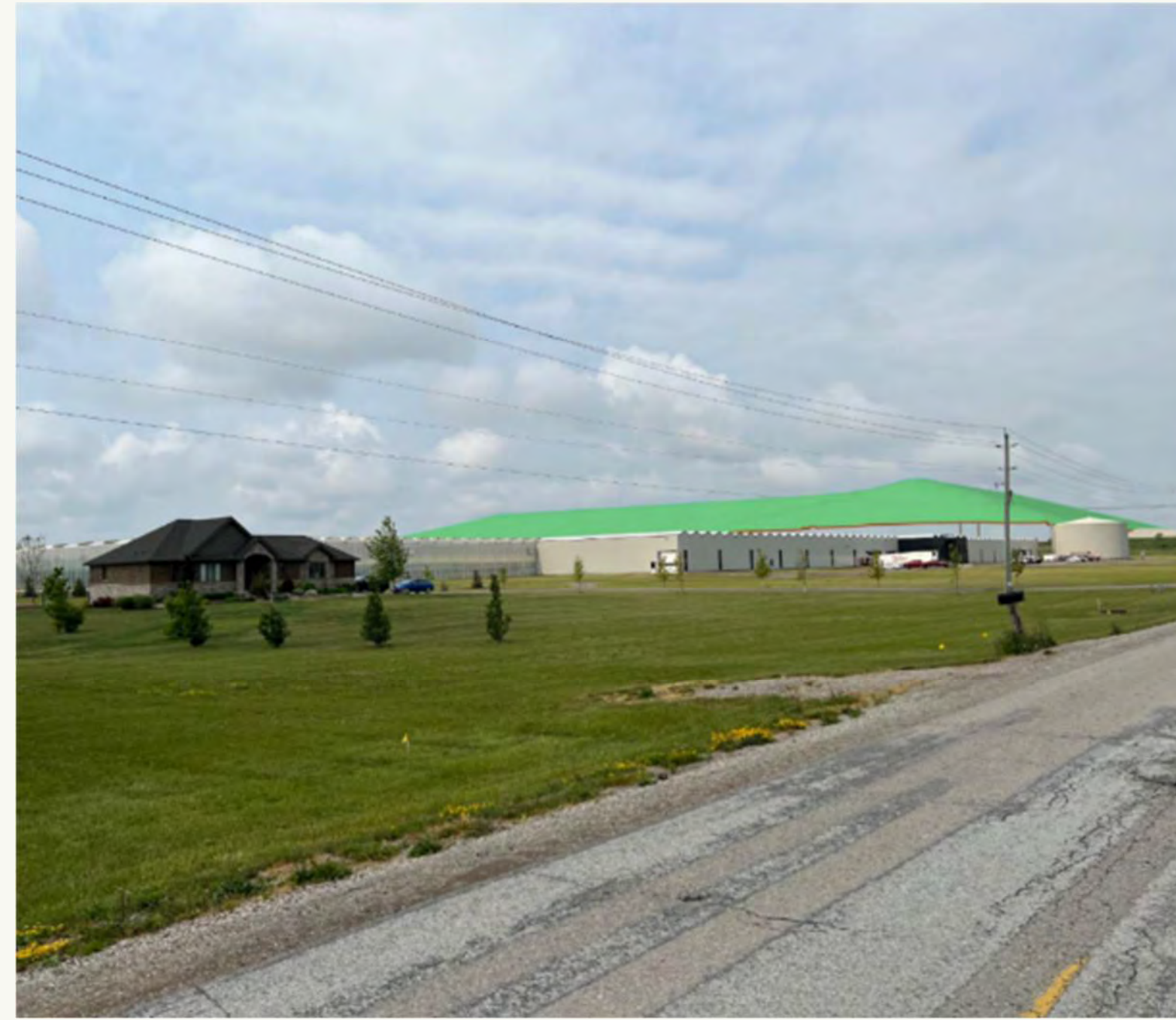
Viewpoint 1 Visible Landfill Area = 41,688 m 2 , index 59.6; effect value = 5. Distance = 700 m; effect value = 4. Horizontal Angle of View = 40°; effect value = 3. VACF = 1; effect value = 5. CEV = 17; high effect.
