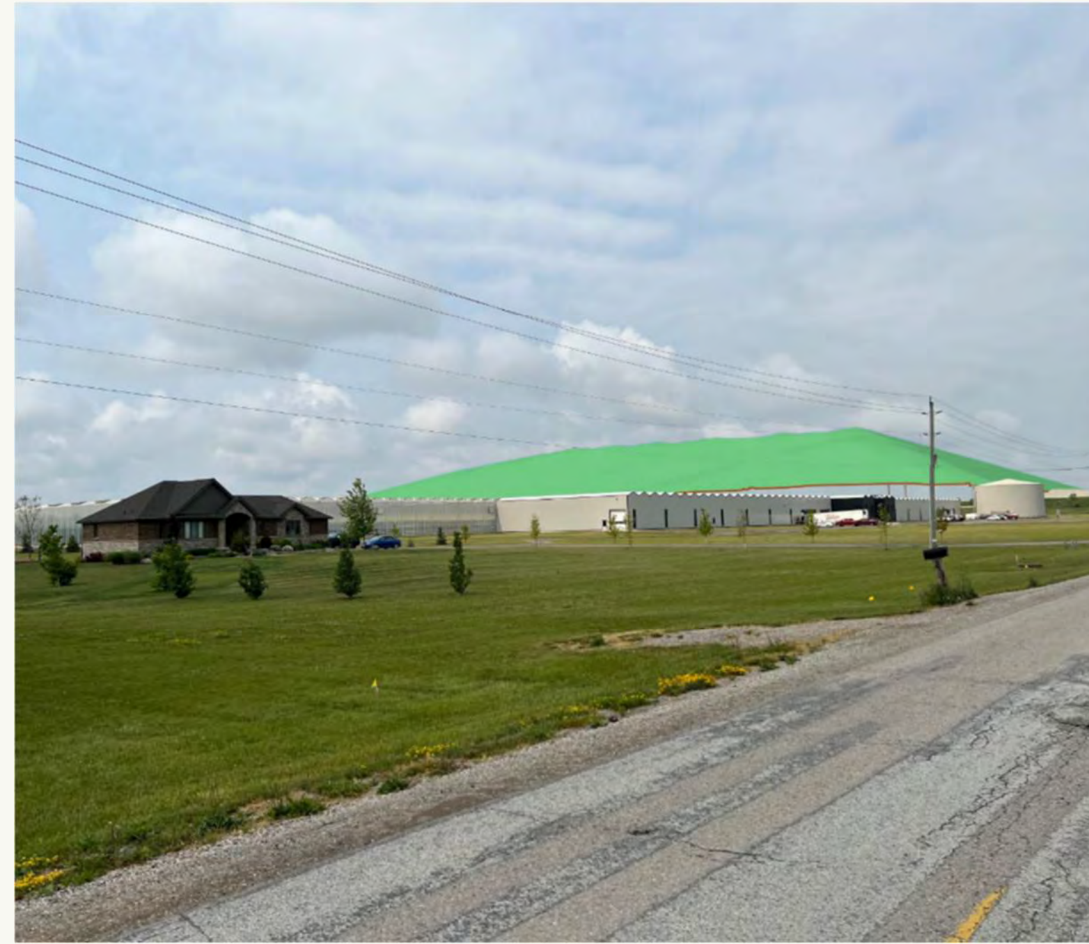
Viewpoint 1 Visible Landfill Area = 63,950 m 2 , index 91.4; effect value = 5. Distance = 700 m; effect value = 4. Horizontal Angle of View = 41°; effect value = 3. VACF = 1; effect value = 5. CEV = 17; high effect.
