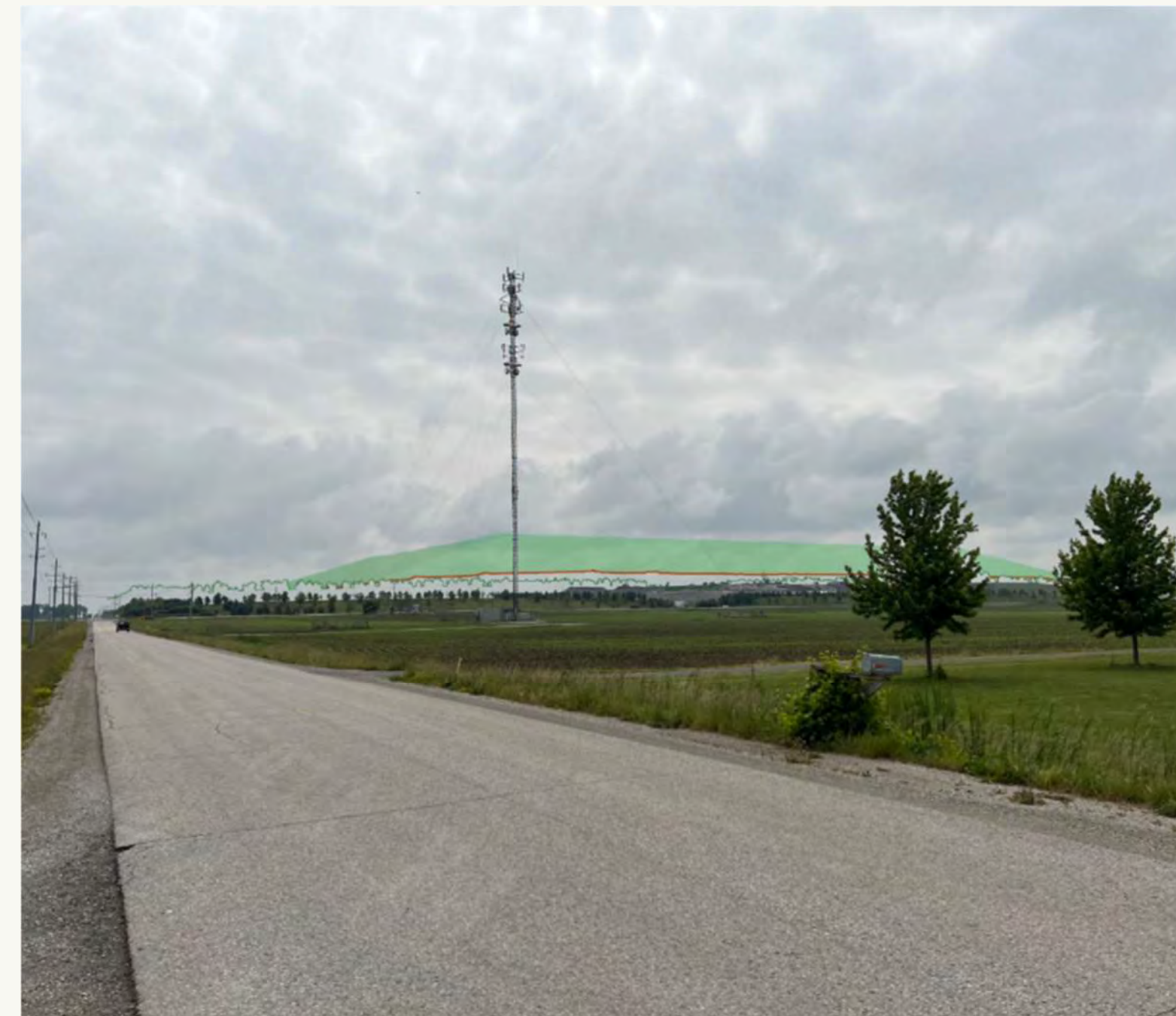
Viewpoint 5 Visible Landfill Area = 40,051 m 2 , index 56.6; effect value = 5. Distance = 707 m; effect value = 4. Horizontal Angle of View = 41°; effect value = 3. VACF = 1; effect value = 5. CEV = 17; high effect.
