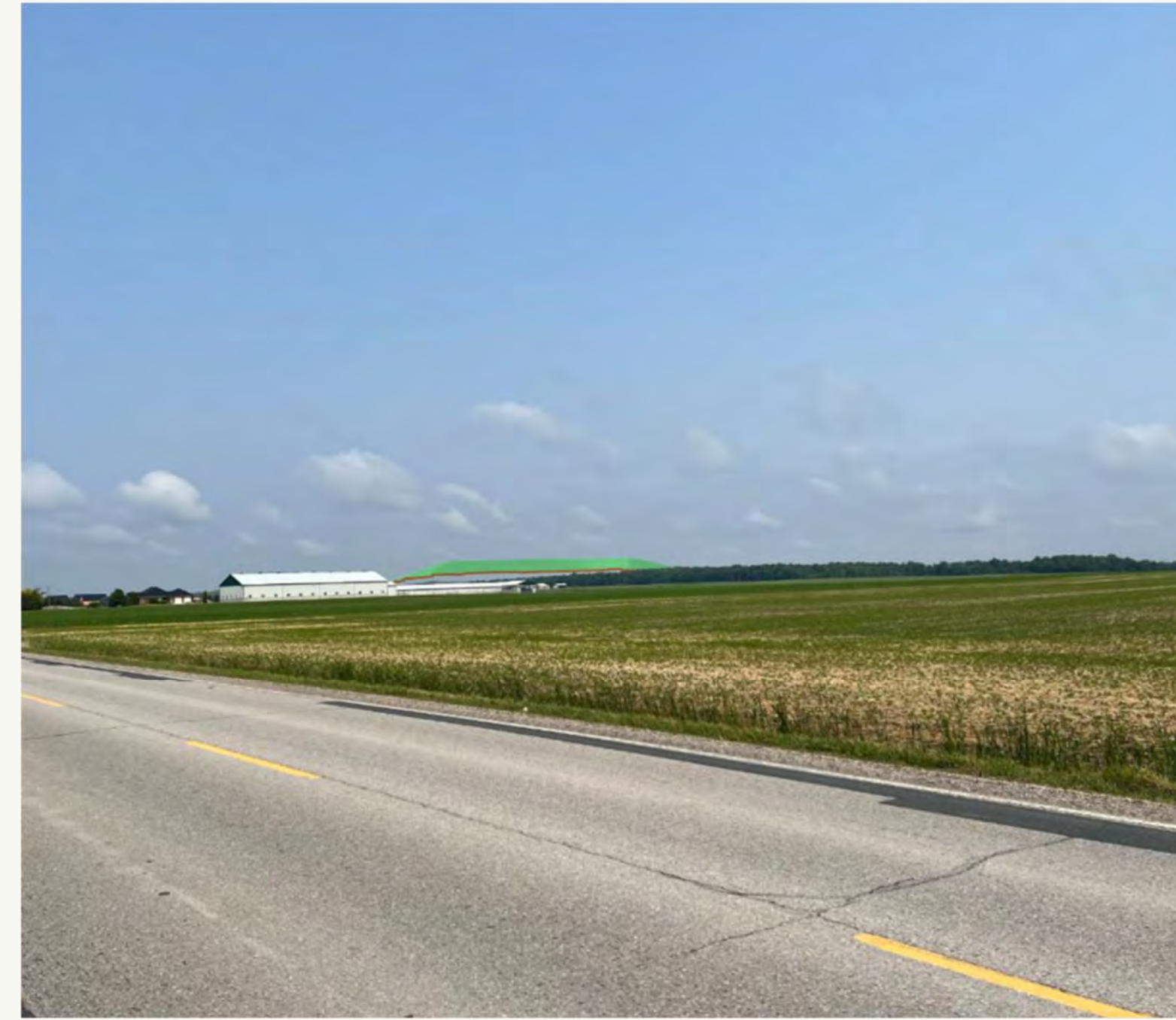
Viewpoint 2 Visible Landfill Area = 40,413 m 2 , index 13.6; effect value = 3. Distance = 2,972 m; effect value = 1. Horizontal Angle of View = 15°; effect value = 1. VACF = 1; effect value = 5. CEV = 10; moderate effect.
