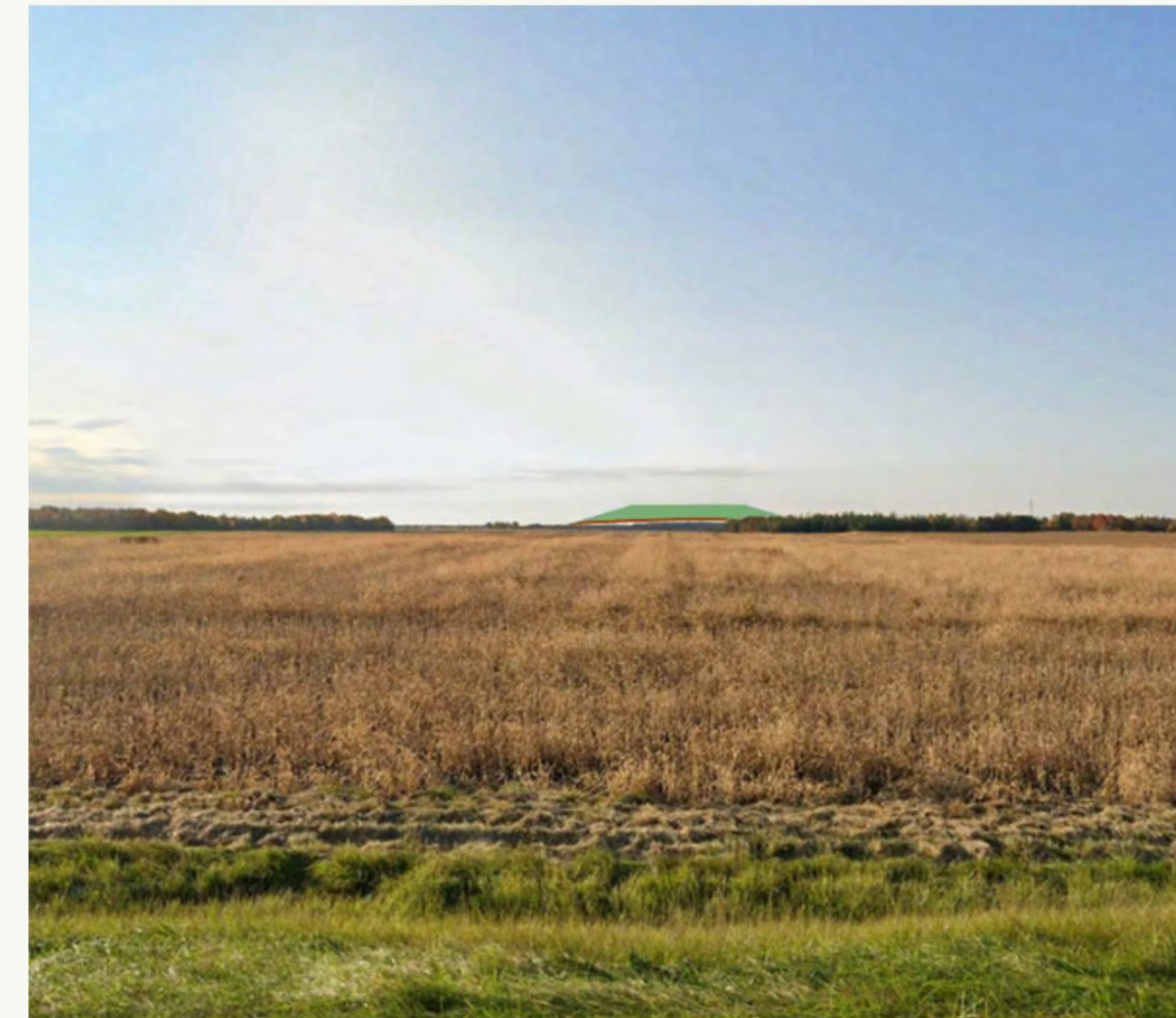
Viewpoint 6 Visible Landfill Area = 19,259 m 2 , index 6.8; effect value = 1. Distance = 2,820 m; effect value = 1. Horizontal Angle of View = 11°; effect value = 1. VACF = 1; effect value = 5. CEV = 8; low effect.
