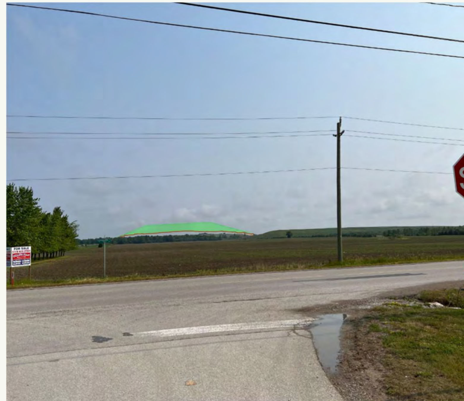
Viewpoint 4 Visible Landfill Area = 21,000 m 2 , index 15.1; effect value = 3. Distance = 1,387 m; effect value = 3. Horizontal Angle of View = 15°; effect value = 1. VACF = 1; effect value = 5. CEV = 12; moderate effect.
