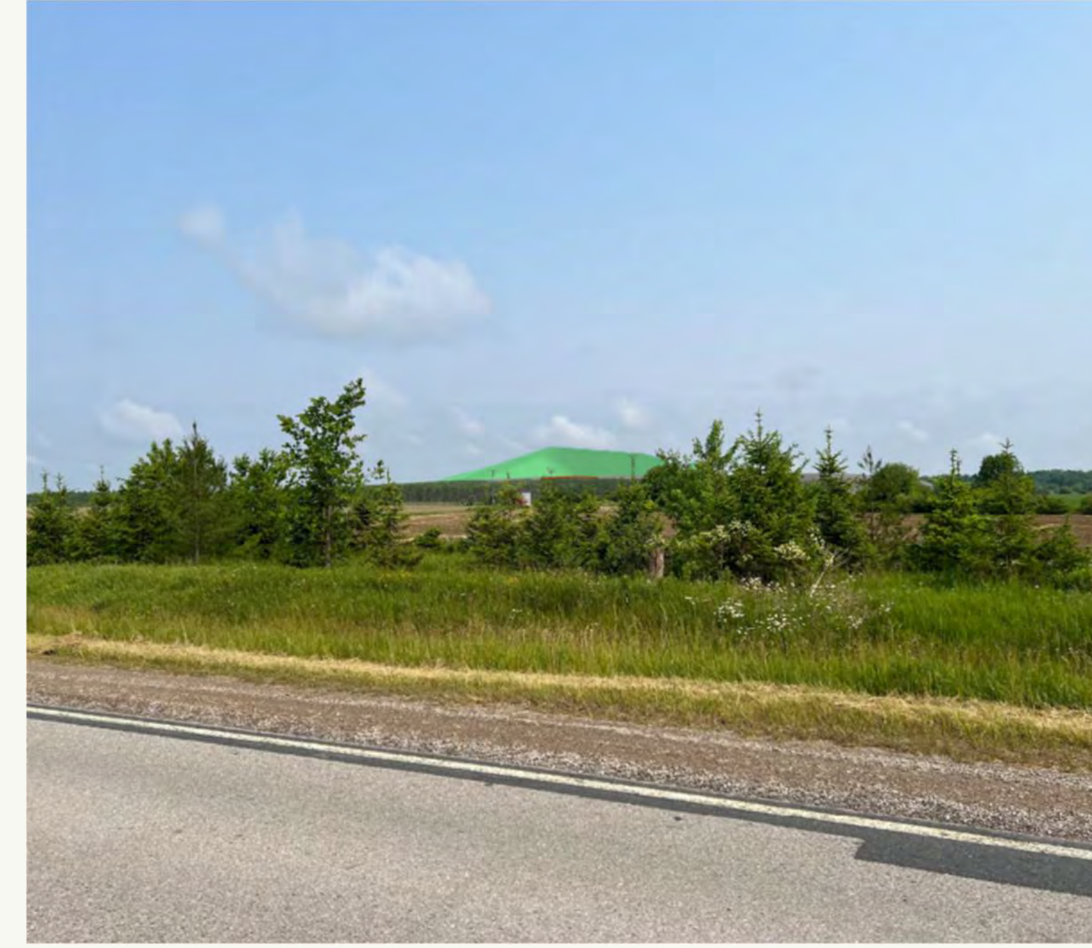
Viewpoint 3 Visible Landfill Area = 61,476 m 2 , index 37.9; effect value = 5. Distance = 1,621 m; effect value = 2. Horizontal Angle of View = 21°; effect value = 2. VACF = 1; effect value = 5. CEV = 14; high effect.
