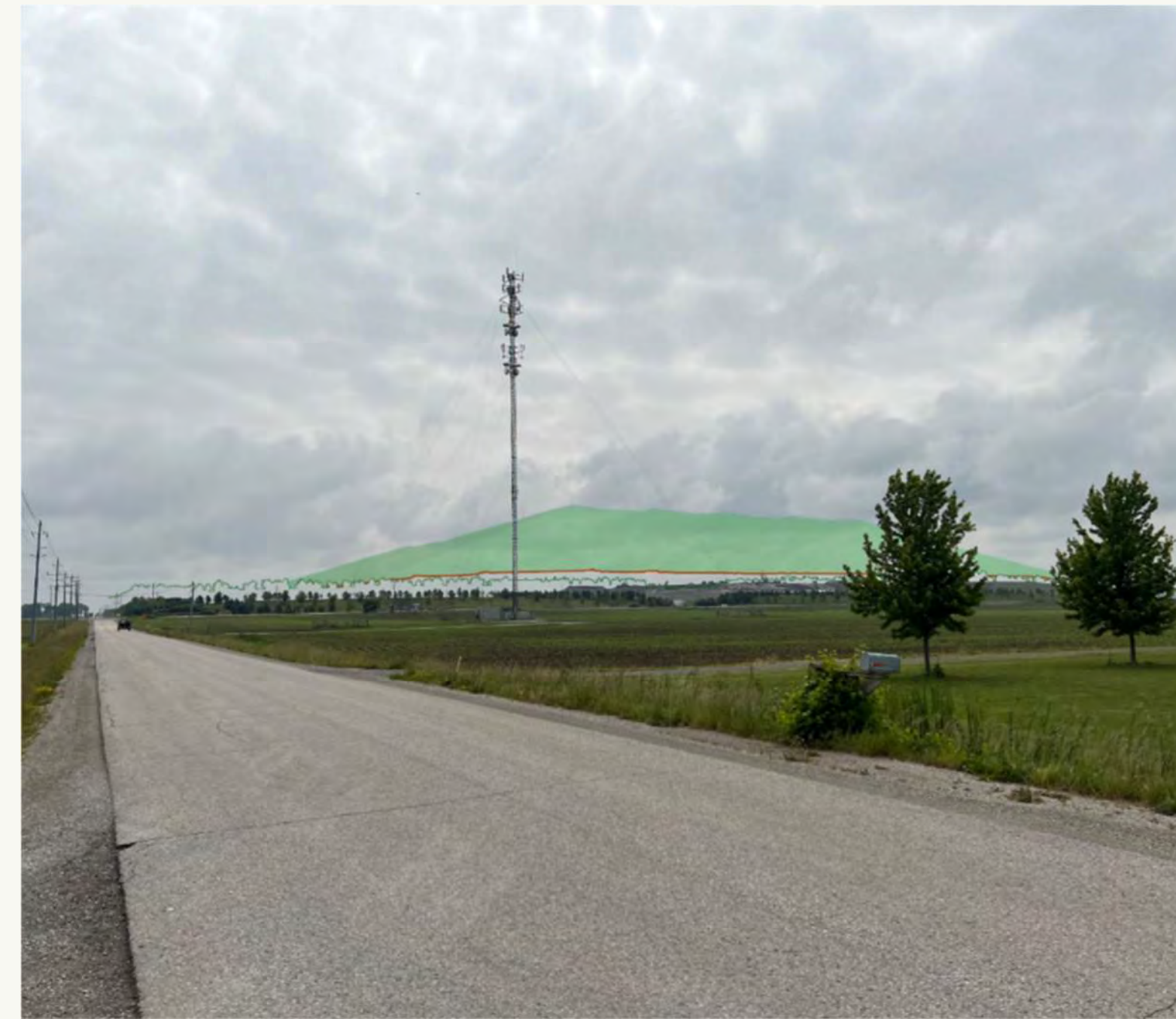
Viewpoint 5 Visible Landfill Area = 60,574 m 2 , index 85.7; effect value = 5. Distance = 707 m; effect value = 4. Horizontal Angle of View = 41°; effect value = 3. VACF = 1; effect value = 5. CEV = 17; high effect.
