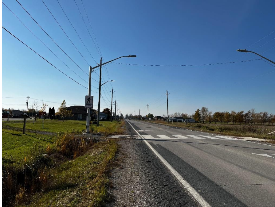
Figure 5-11. Confederation Line, looking west
