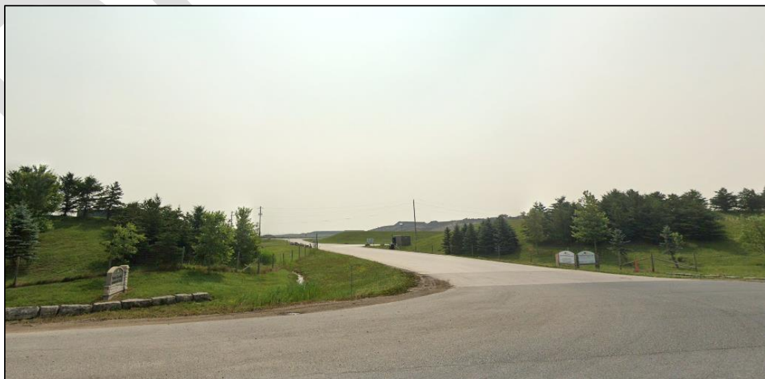
Figure 4-15. Looking east towards the TCEC Entrance on Nauvoo Road
