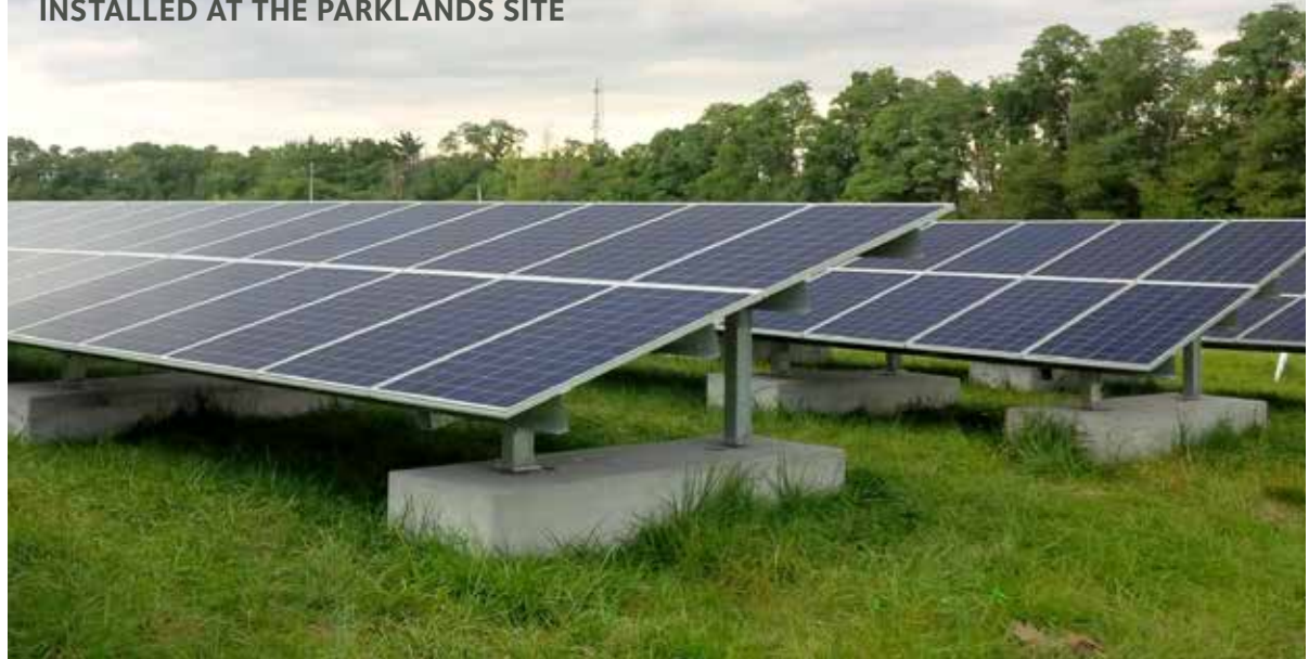
RACKING FOR THE SOLAR PANEL SYSTEM BEING INSTALLED AT THE PARKLANDS SITE
